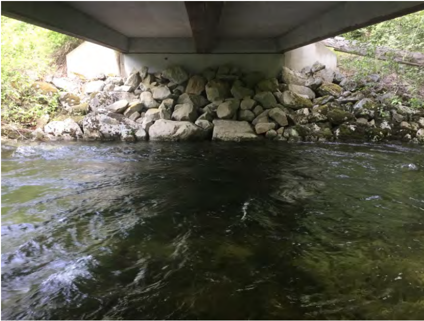
Left Bank Abutment when facing downstream
