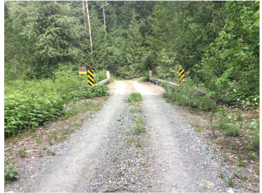
Approach from Right Bank when facing downstream
