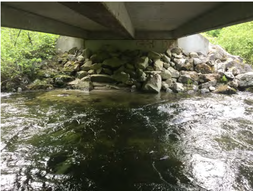
Right Bank Abutment when facing downstream
